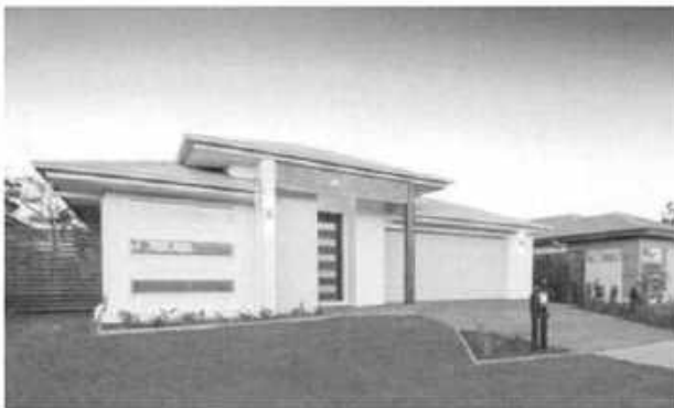
STREET FRONT DESIGN: PROVIDING AN ARTICULATED AND QUALITY DESIGNED FAÇADE ENHANCES BOTH THE DWELLING ITSELF AND ITS SURROUNDING STREETScape
