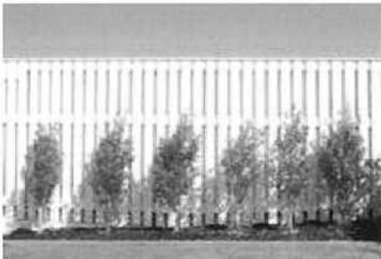
DIAGRAM C: GOOD NEIGHBOUR FENCING Fencing is to be timber, 1800mm high and 100% solid. Must be constructed of A grade CCA treated pine timber palings (3 rails, palings both sides and timber posts) with a continuous capping.
