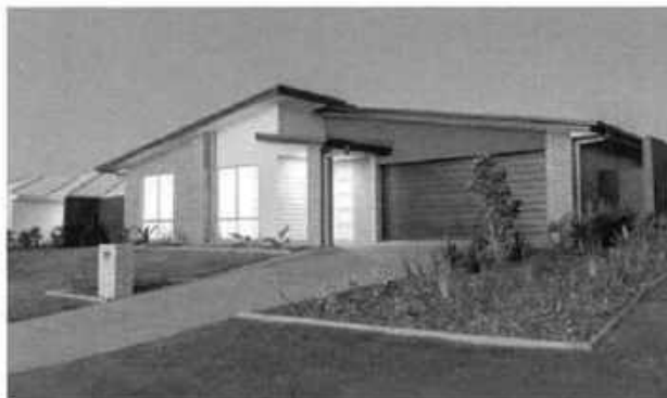
LANDSCAPE REQUIREMENTS: USE OF NATIVE TREES THAT ARE RESPONSIVE TO THE REGION'S CLIMATIC CONDITIONS.
